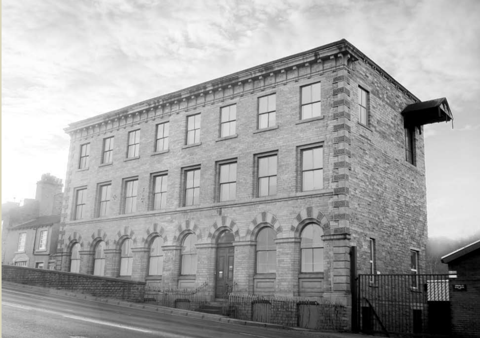
The original Bankfield Mills – built in 1829 and the home of W.T. Johnson & Sons since 1910. The building is still in use today within the current W.T. Johnson & Sons site.
